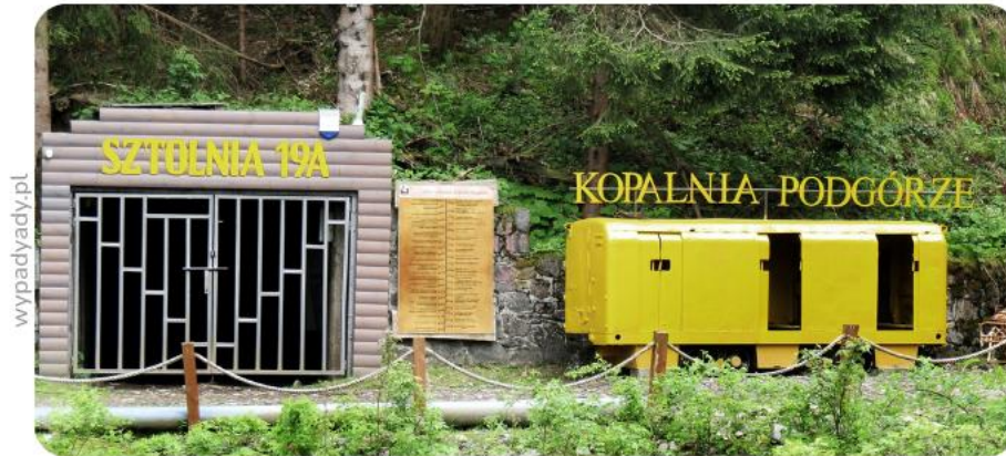
Entrance to adit no. 19a in the Podgórze mine.
